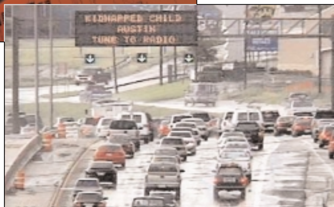
SwRI software engineers have designed and deployed dynamic message sign (DMS) subsystems in many traffic management centers (TMC). These subsystems integrate different DMS protocols to give TMC operators a seamless operation in displaying to the public messages such as Amber Alerts.
